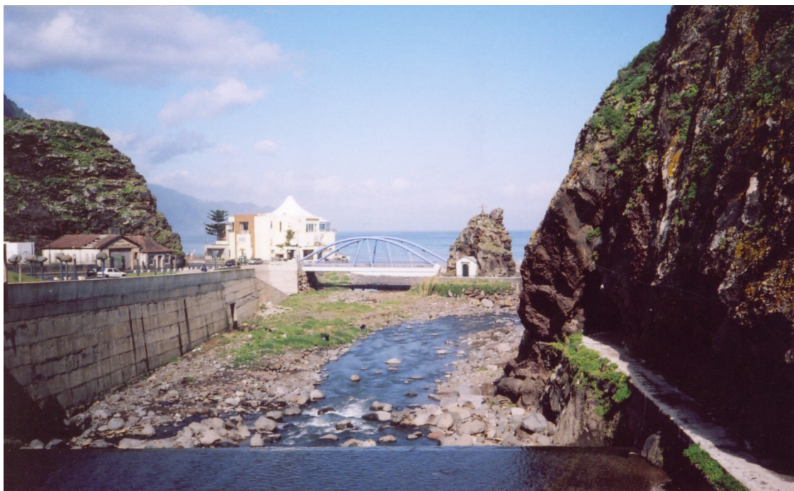
Figure 2. State of conservation of São Vicente main watercourse river mouth.
